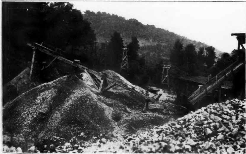
Chute for Gravel from Hummer Screen
